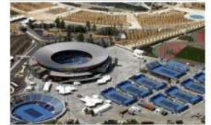
OLYMPIC TENNIS CENTRE, Potiroopoulos Arch (2004)
